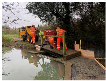
We are pleased to advise that the repairs to the spillway were carried out by Rutland County Council contactors in mid-December. These repairs were originally scheduled for mid-November but the snow delayed the work. Rather than holding back water when the canal is in flood, the design is to allow excess water to flow over the top of the spillway without eroding the foundations of the spillway bridge.
