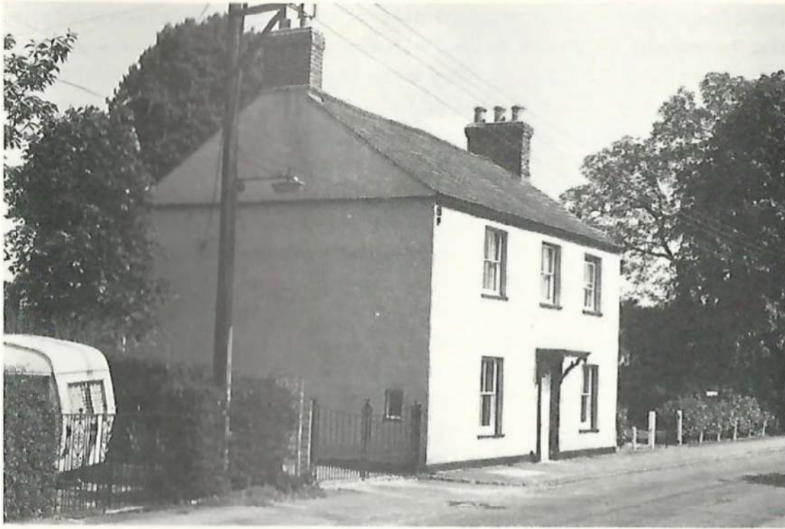
The former Boat Inn, Ashwell Road, Oakham in 1983. Note the small window at the side, presumably to serve ale to persons using the wharf on the canal at the rear
